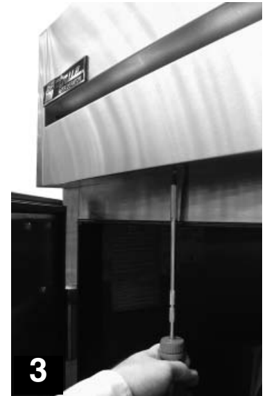
3 Three Door Freezer unit (Rainshield Removal / bottom screws)
