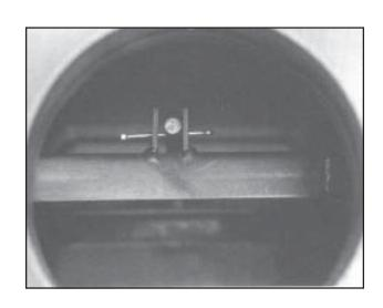
16. Next working through the flue hole behind furnace, line up rod between the two posts on the sliding smoke damper. Then line up the three (3) holes for cotter pin insertion, this procedure will test your patience. It's helpful to have a flashlight and another person positioning the rod.
