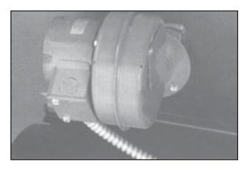
3. Attach the draft fan to the back of the weld on the throat (2" throat hole with 3 mounting holes). It's best to use the self tapping screws without the draft fan to establish threads then mount blower. The electrical box on the blower should be facing downward. Draft fan air intake cover should be set at a 20% opening, about 1/2" opening.
