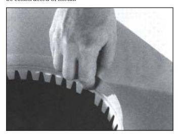
**Installing collar to top:** To install hot air attaching collar, simply bend all tabs right angle under shroud. This may be possible with thumbs, if not, remove top and use small hammer.
