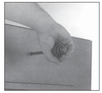
13. Installing front and rear cast baffles, heat plates. NOTE: Grate frames and brick will slide forward and backward to allow baffle to fit. Install front cast baffle using two (2) 5/16 bolts, nuts & washers (7/16 wrench will be needed). Place the side of the baffle that has the two ribs against the front weld of the firebox. Do not tighten bolts yet. Place the rear cast baffle to the back of the firebox but do not attach the bolts at this time.
