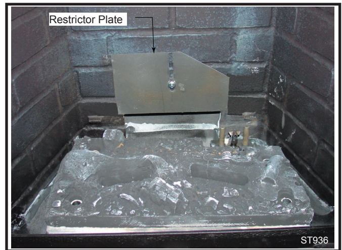
Fig. 9 SDDVT/SDDVTC restrictor plate.
