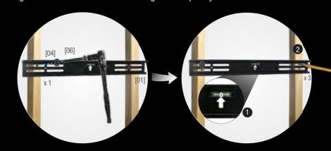
Secure the remaining lag screws to wood studs securing all four tightly.
