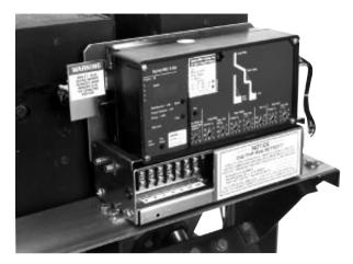
A. Mount the Trip Unit / Aux. CT Module Assembly to the Trip Unit Mounting Platform as shown, using the (4) .250-20 × .750" bolts, (8) flat washers, (4) lock washers, and (4) nuts supplied.
