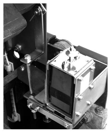
A. Mount the DTA Mounting Bracket to the right Breaker side panel, as shown, using the holes drilled in Step 5 A and the (2) .312-18 × .750" screws, (2) flat washers, (2) lock washers, and (2) nuts provided.
