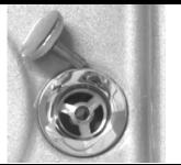
Picture, of drain plunger removed, shown for cleaning reference.
