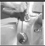
Step 1: To remove the chrome drain handle, loosen the set screw in the slot on the drain handle and slip off chrome handle from chrome handle post.
