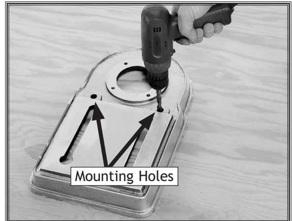
Figure 17. Using holes as a drilling guide.
