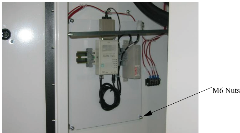
Figure 1 Panel with Four M6 Nuts
