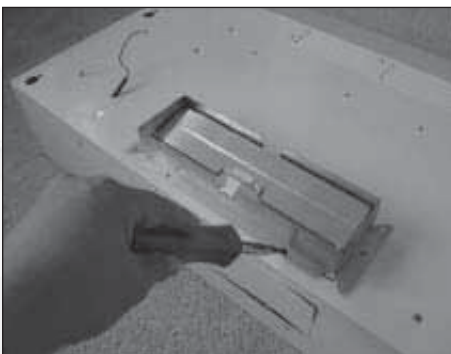
5. Attach the 3 1/4" X 10" starting collar with damper to the duct opening you exposed.
