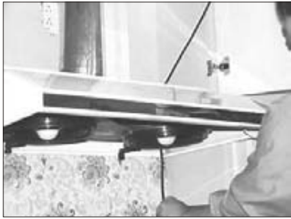
11. Pull electrical supply wire through drill out or use #14 grounded wire for receptacles (not supplied).
