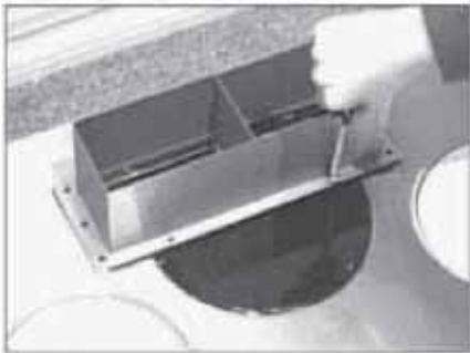
3. Mount the 3-1/4"x10" starting collar on top of transition piece with remaining screws.
