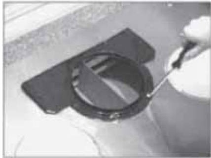
1. Remove pre-mounted 7" transition adaptor or duct opening.
