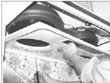
14. Reinstall bottom splash shield by first fastening 3 rear screws, (do not tighten all the way).
