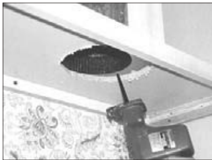
4. Cut out cabinet base opening if necessary.
