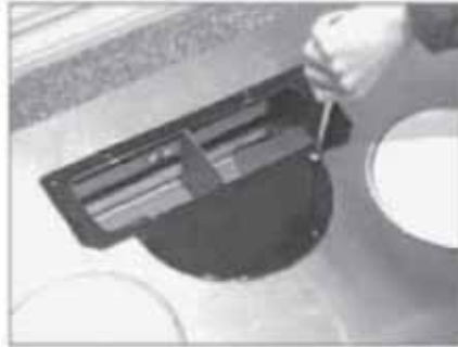
2. Place rectangular transition adaptor as shown by first installing 4 screws on half round section.
