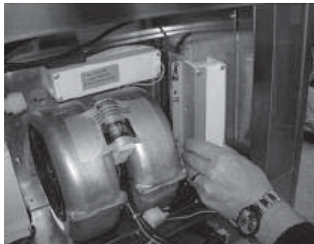
3. Position capacitor box as shown.
