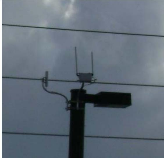
In this example we see the Canopy backhaul radio with its antenna pointing towards the MOTOMESH Duo device. This results in strong interference.
