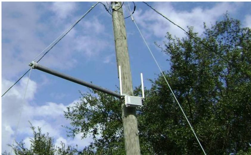
In this example we see the MOTOMESH Duo device mounted with its antenna next to a steel pole. This results in antenna pattern distortion.
