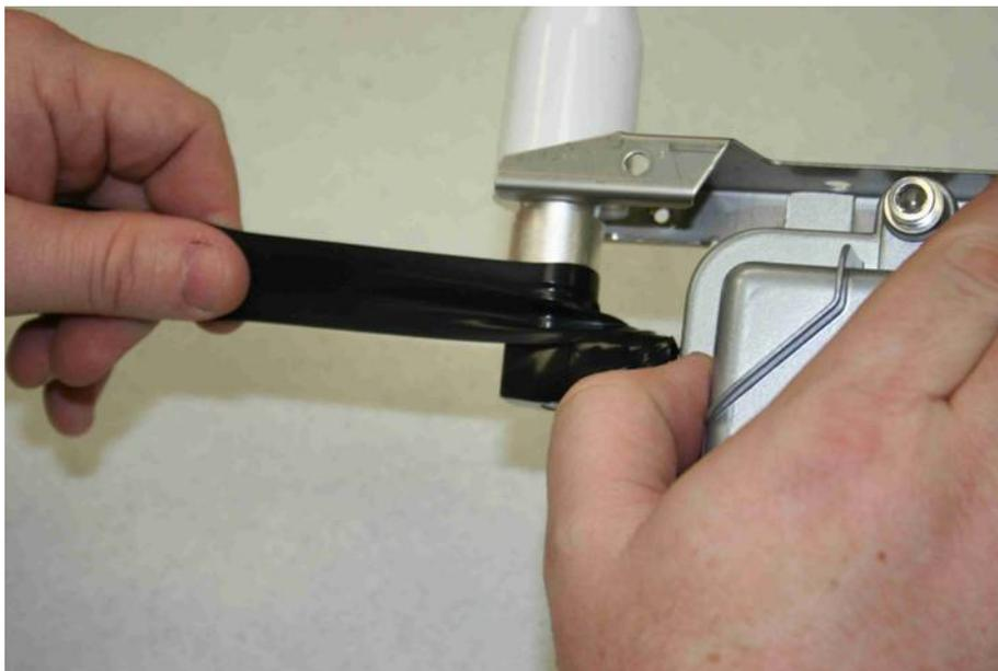
Figure 4-16 Use electrical tape and cover the weatherproof tape
