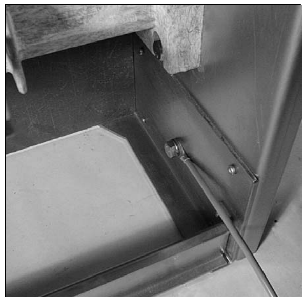
Fig. 14 Installation of Ground Wire
