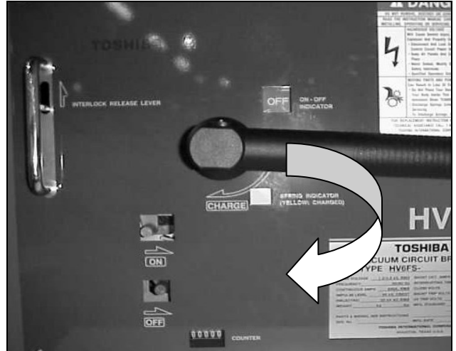
Fig. 25 Preparing to Manually Close Breaker
