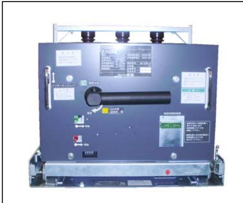
Figure 11 Attach the handle provided with the unit to the handle shaft. Check to make sure that the handle has been securely connected to the shaft (small screw M5).
