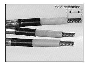
2.6 Remove cable insulation from conductors ends of both **Cable X** and **Cable Y**.
