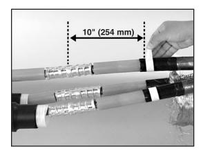
4.5 Apply red compund on cable insulation, making certain to fill in edges of cable semi-cons.
