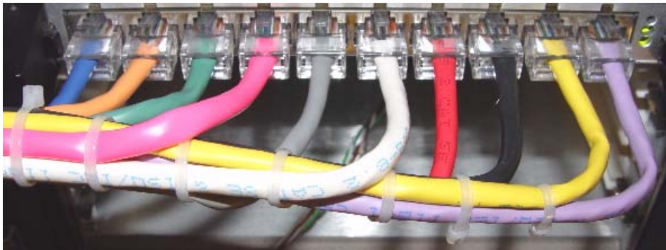
FIGURE 1-19 FE10 RJ45 Connector Dressing
