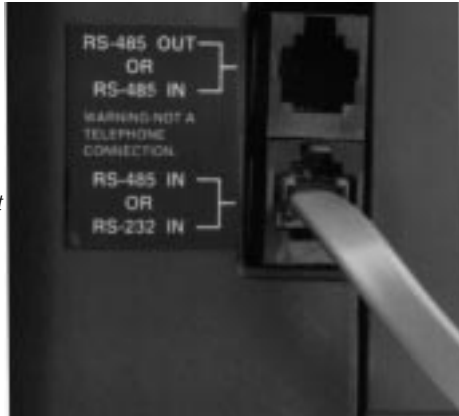
Figure 15: Data Receiver cable installation.
