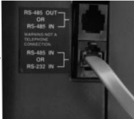
Figure 20: Data Receiver cable installation.
