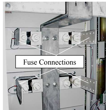
Figure 5-10 Fuse Bay Connections
