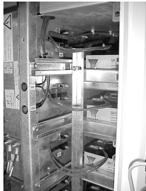
Connect all battery drawers to the terminal on the left side of the column
