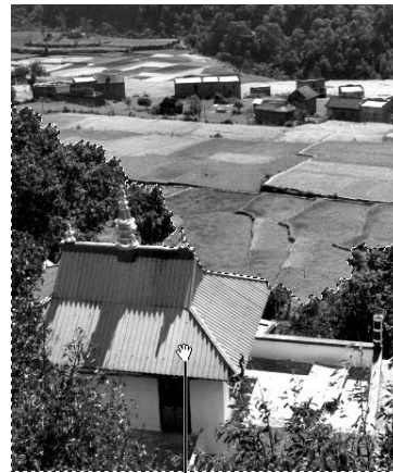
The building was moved to cover the sheds.
