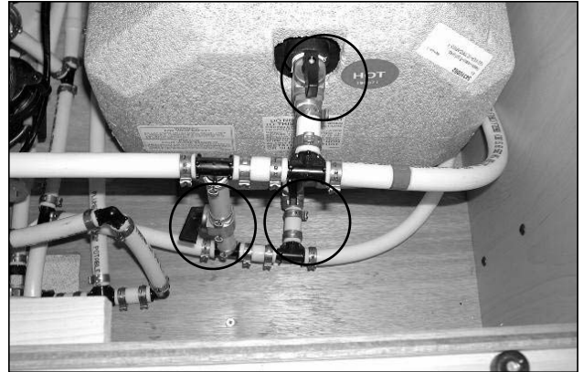
Picture G-P14: Summer mode valve positions.
