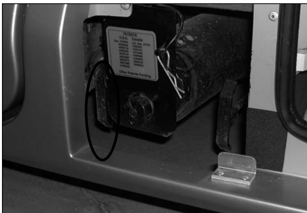
Picture B-P43: Exterior fresh water drain valve, (170 model).
