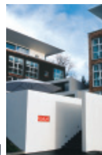
The BODUM headquarters in Triengen, Switzerland, was designed by the the BODUM Design Group from 1996 to 2000. The 27,000 sq.ft. building, designed around its cafeteria, makes the flow of communication easy for the 50 people working there.
