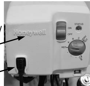
Spark igniter/flame sensor wire
