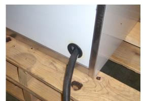
4. Remove the brass caps on the sides of the junction box and insert the power cables.
