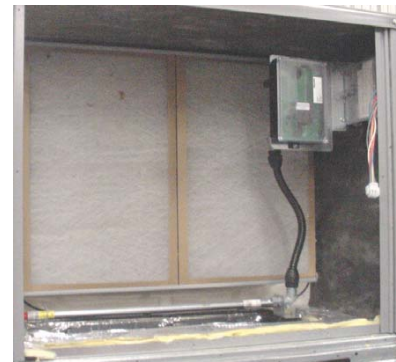
Fig. 22 - Return Air Sensor Operating Position
