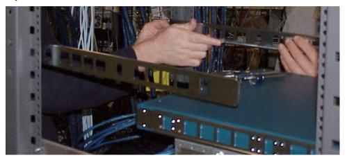
Figure 1-3: Holding Rack Bracket Against Inside of Rack
