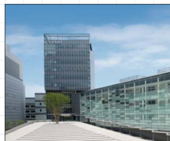
Headquarters and Technical center building
