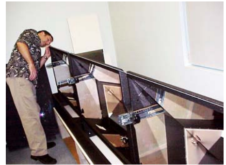
Using string to see that the row is straight
