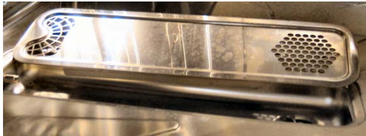
Drain Cover and Drain
