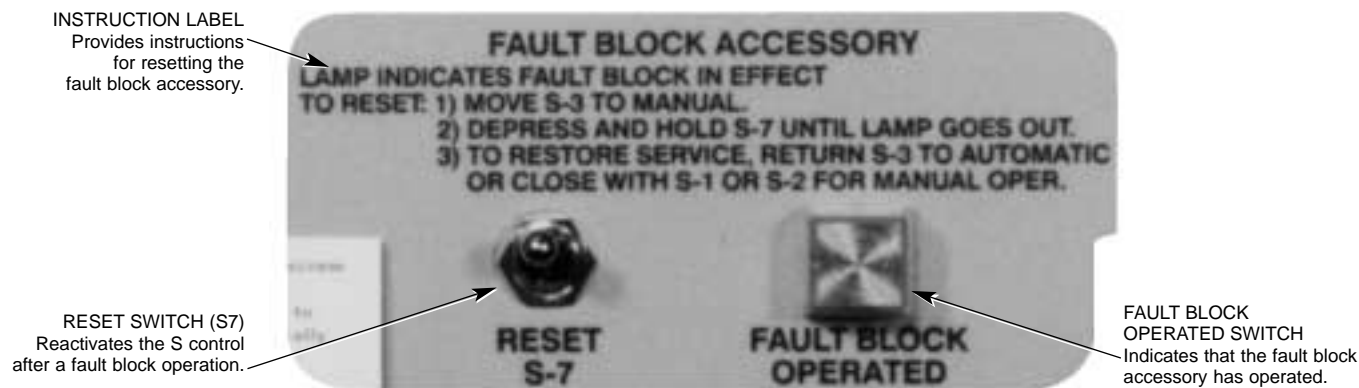
Figure 19. Fault block accessory controls and operating instructions plate.
