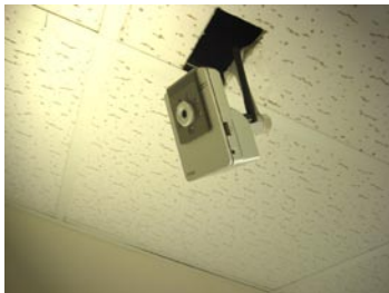
On the ceiling
