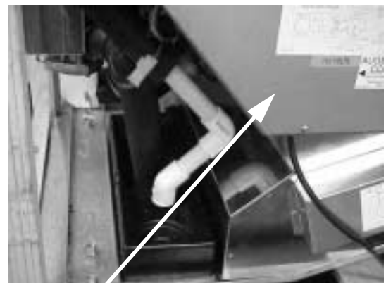
Remove Insulation from Drip tray Drain Line Assembly
