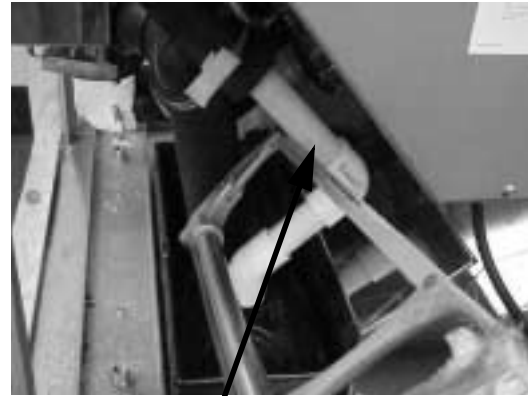
Cut PVC Drain
