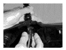
Slide one dash adapter nut (F) over supply lines and thread onto adapter until seated on the bottom surface of dash. Tighten using moderate force. Do not over tighten.
