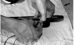
9. Screw the mounting plate into the mount using the two previously removed 3/8" #6 screws. This will secure the LED assembly into the housing. You are now ready for reassembly.
