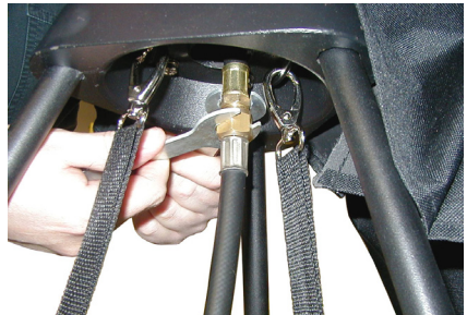
Figure 11 - Attaching Regulator Hose to Burner Fuel Line
