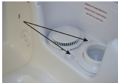
1 1. Bleeder Valves Figure 12. Bleeder Valves
