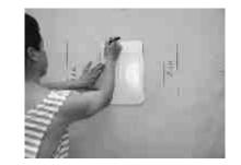
) Using a drywall saw, cut out the opening.
