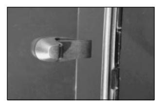
Squeeze the latch in the center of the window and slide the glass to open it.
