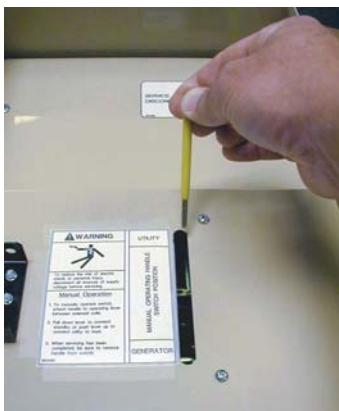
Figure 3.1 — Actuating Transfer Switch
