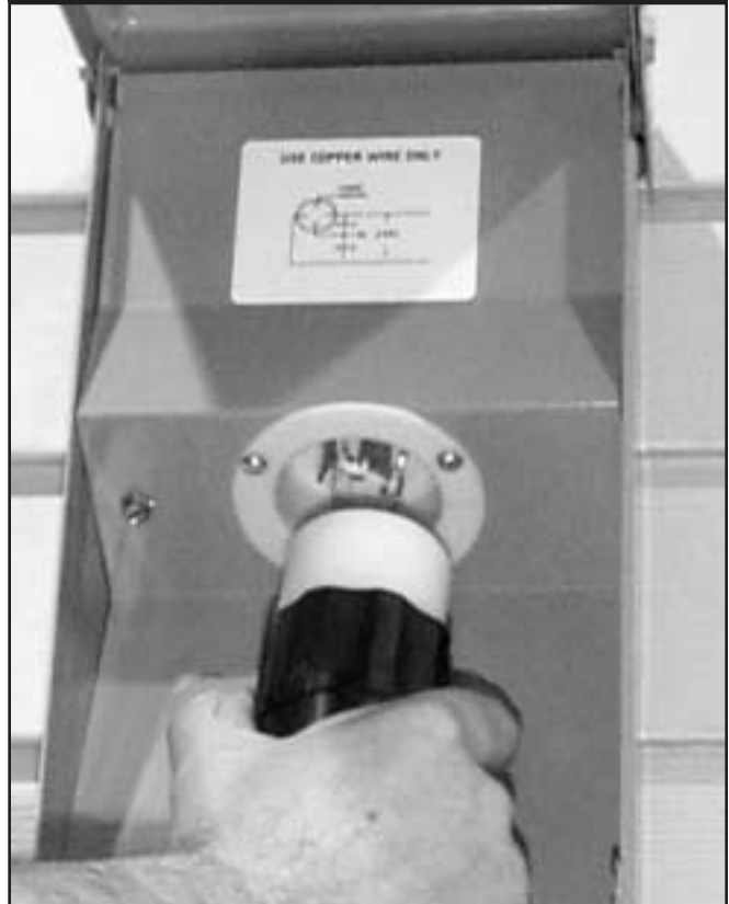
Figure 19 — Connection Box Connection
