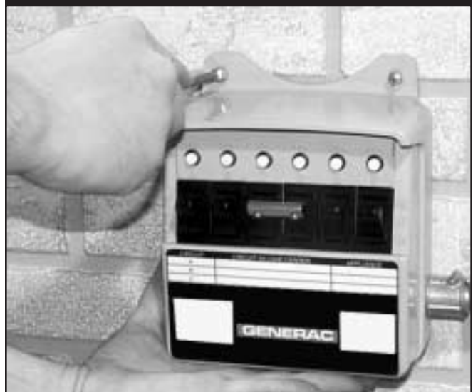
Figure 4 — Anchoring Load Manager™ Switch
