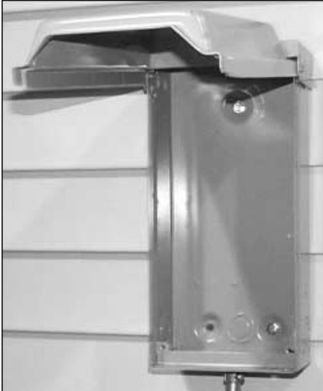
Figure 13 — Connection Box Installation
