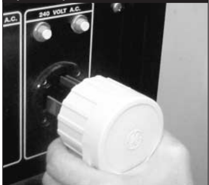
Figure 20 — Align Connector at Generator
