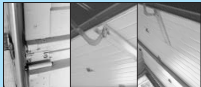
FIG. 2-6 Examples of door bracing.
