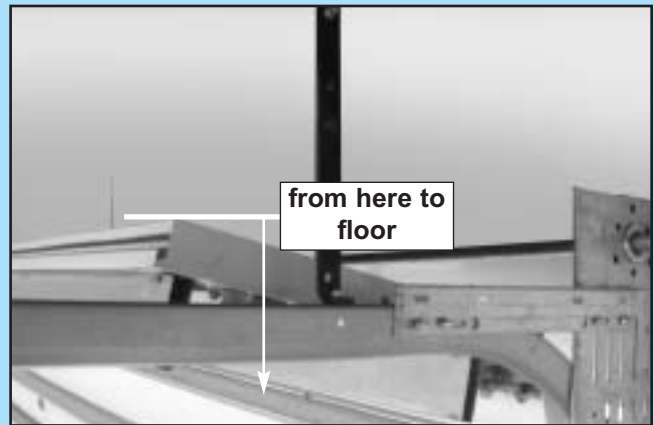
FIG. 2-1 Finding highest point of travel (sectional).
