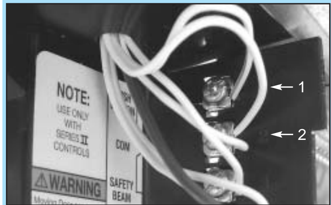
FIG. 5-1 Terminal attachments at power head.
