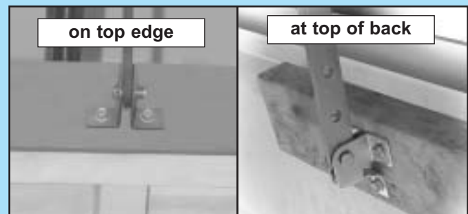
FIG. 2-7B Mounting door Bracket (one-piece).
