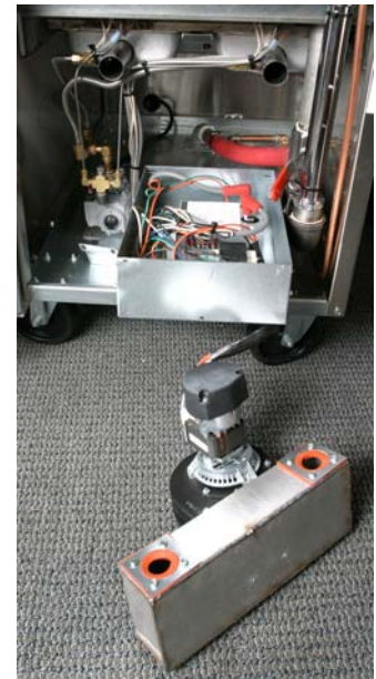
Blower and plenum removed
