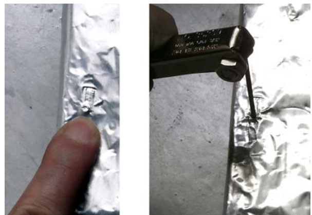
Fig. 10, 11: Find the set screws under the foil insulation and push through with an allen wrench.
