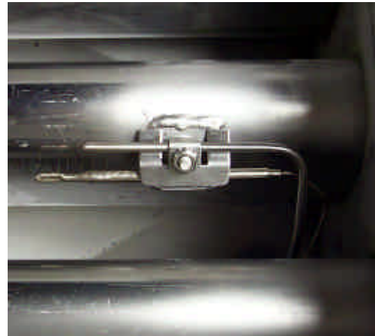
Typical high-limit/sensor probe locations and mounting hardware.
