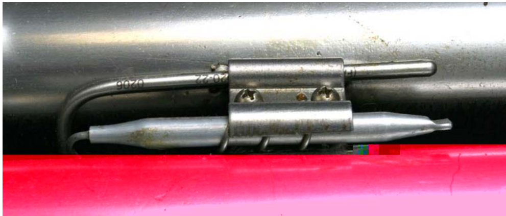
Typical high-limit/sensor probe locations and mounting hardware.
