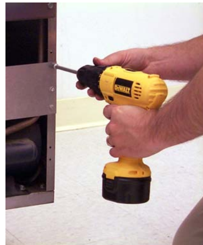
Removing gas manifold shield.
