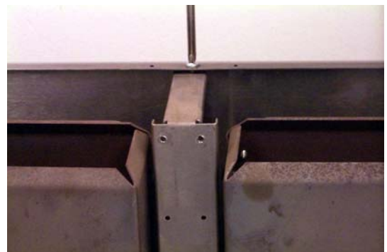
Removing brace holding back panel to flue cap.
