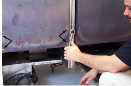
Removing bolts (arrows) securing flue to frypot.
