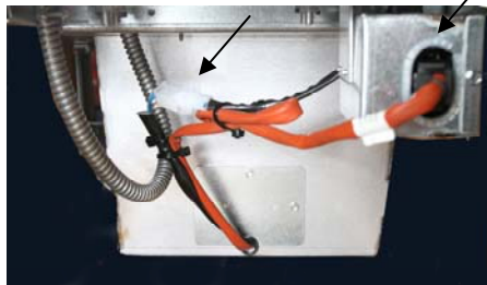
Figure 3: Attach the two-pin white connectors and plug the black connector into the utility box as shown.
