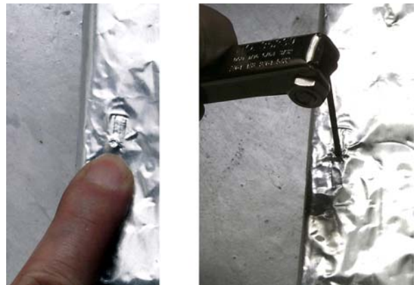
Fig. 10, 11: Find the set screws under the foil insulation and push through with an allen wrench.
