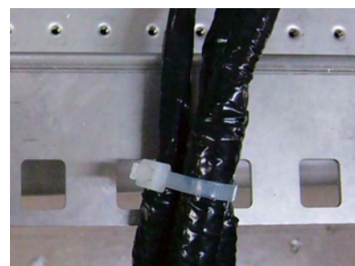
Fix cables to post with cable tie
