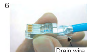
Insert the cable into the modular plug so that the folded part of the shield enters into the plug housing. The drain wire should be located on the tab side of the plug.
